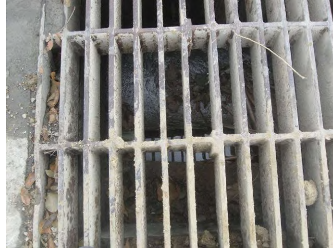
Close-up of storm drain, with view of sheen on water in drain sump
