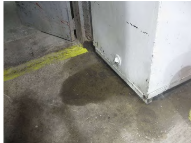
Close-up of release from hydraulic oil AST - Lawson space
