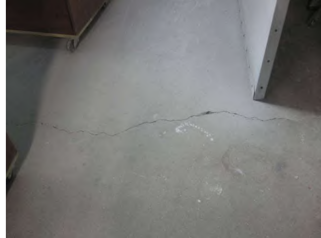
Crack on concrete by paint booth (Srbecky tenant space)
